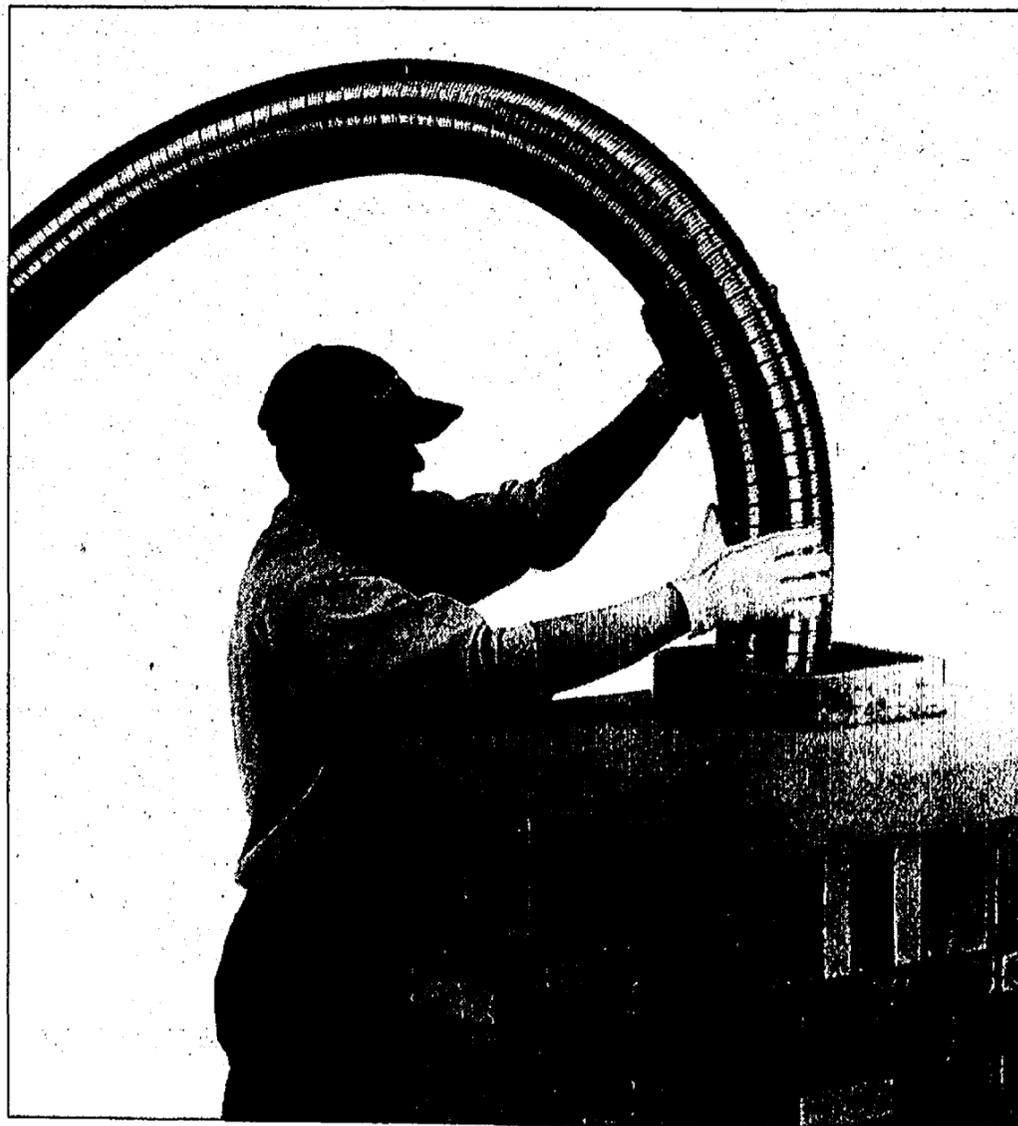
Installing a stainless steel chimney liner can reduce the risk of chimney fires or carbon monoxide poisonings from deteriorating masonry chimneys.
